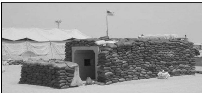
Figure 8-12. Example improvised bunker using concrete culvert sections
