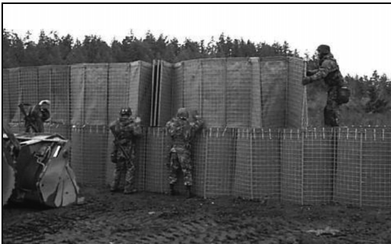
Figure 8-11. Wire and fabric container revetment
